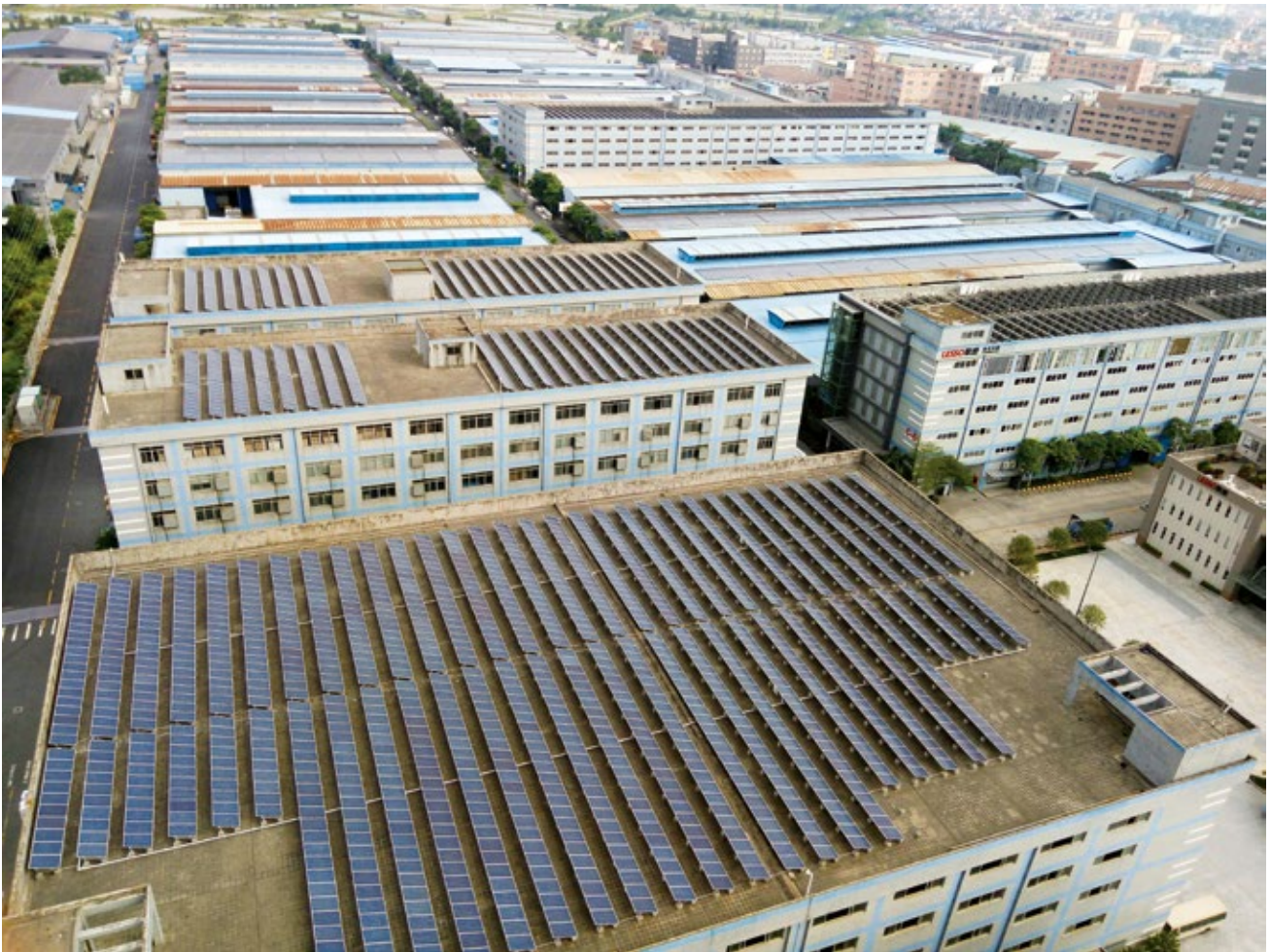
Solar PV Panels on the Roofs of Lesso Plants 聯塑廠區屋頂太陽能光伏板
