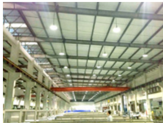
Conversion to LED lighting in the headquarters 總部 Led 改造
